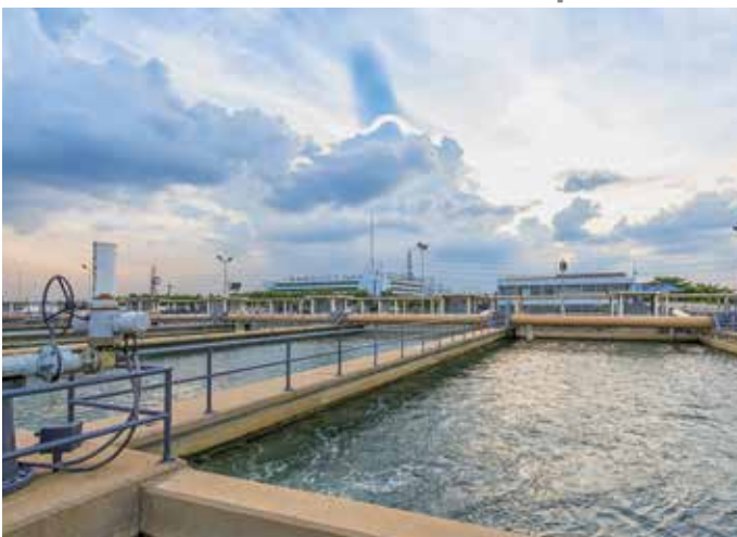
Waste Treatment Plants - Station d'épuration
